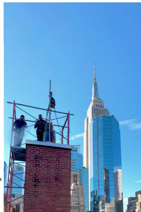
Phase 5 End polymerization and cut of the liner. Take out the internal plastic bag. Seal with epoxy putty on the rim of the cuts.
